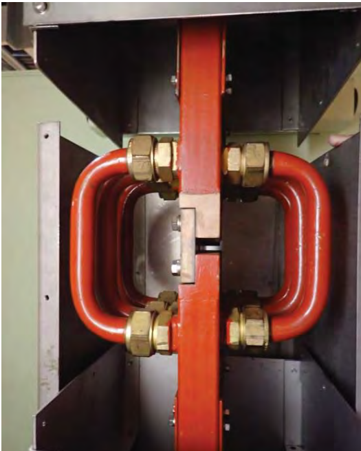
点検箇所①
