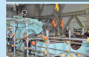
Dismantling of turbine generator
