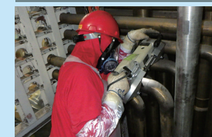
Dismantling of pipes above the reactor
