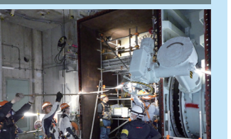
Dismantling of condenser
