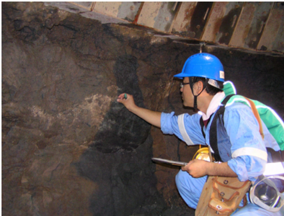
Shaft wall observation
