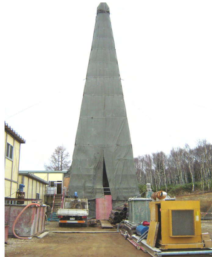
Borehole investigation at the HDB-11
