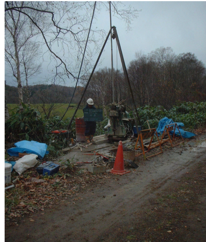
Example of borehole investigations
