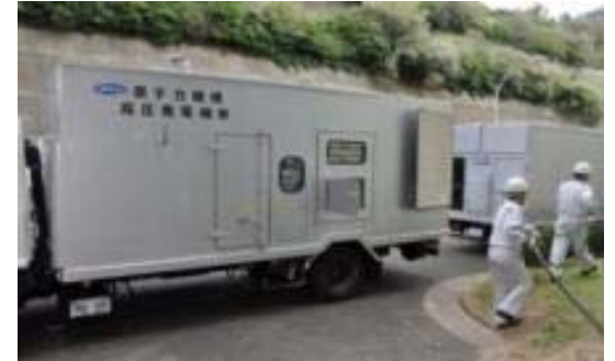
Training of connecting work to emergency power supply car
