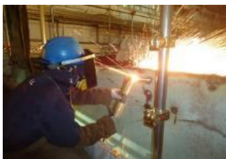
Cutting using gasoline
