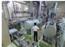
Verification of rationality of the dismantling procedure
