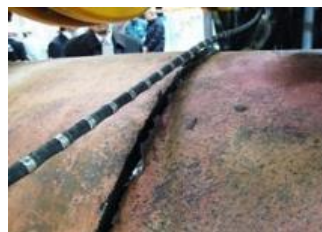
Cutting with diamond wire saw
