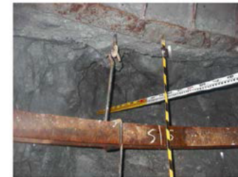
Spalling at shaft wall
