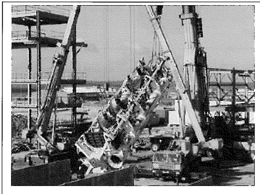
Figure 9: Assembling of the sinking platform
