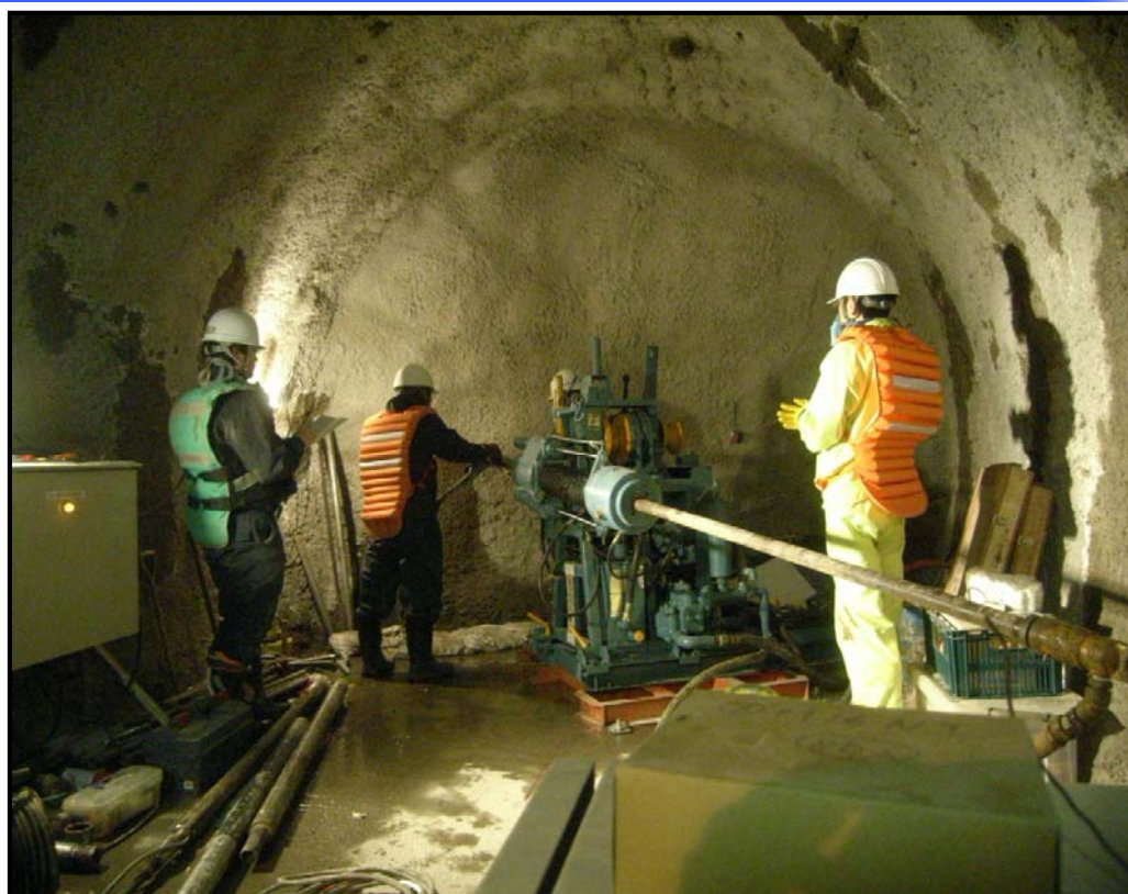
換気立坑：深度140m
