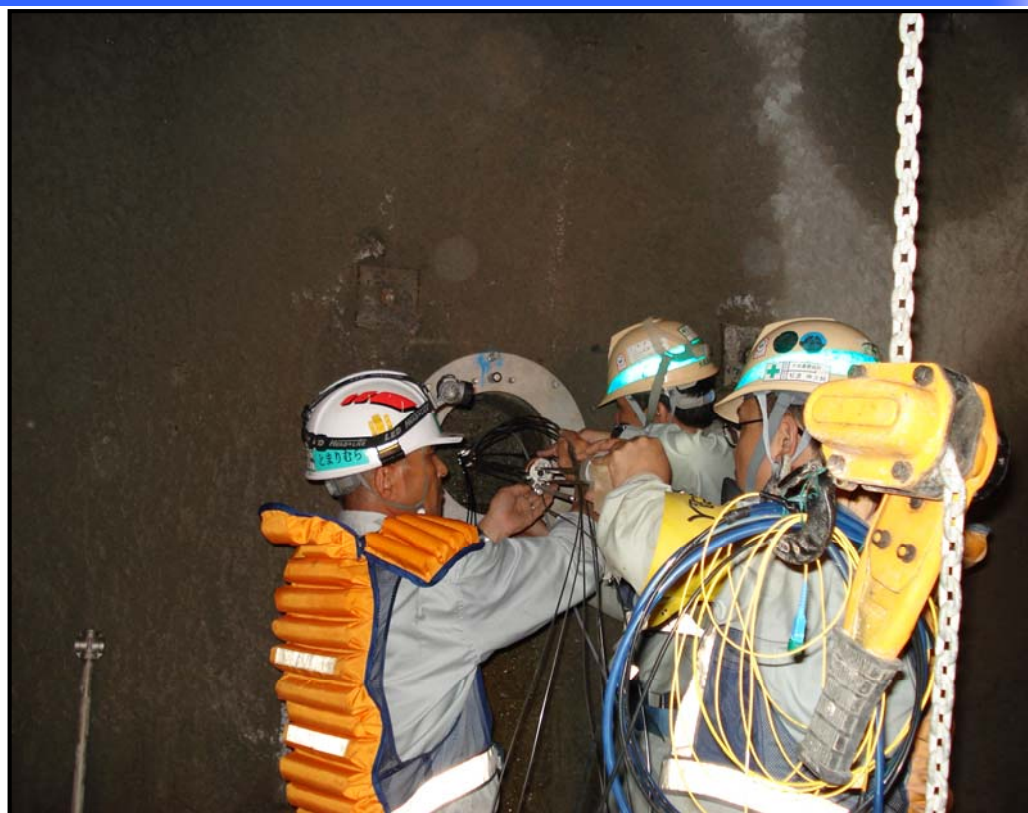
換気立坑：深度70m
