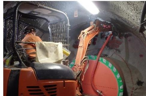
Removal of gap filling material by Auger drilling
