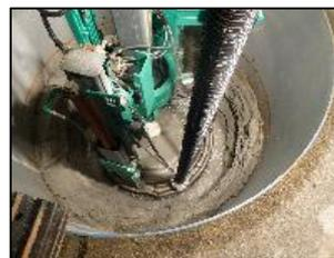
Removal of the buffer material by saline water
