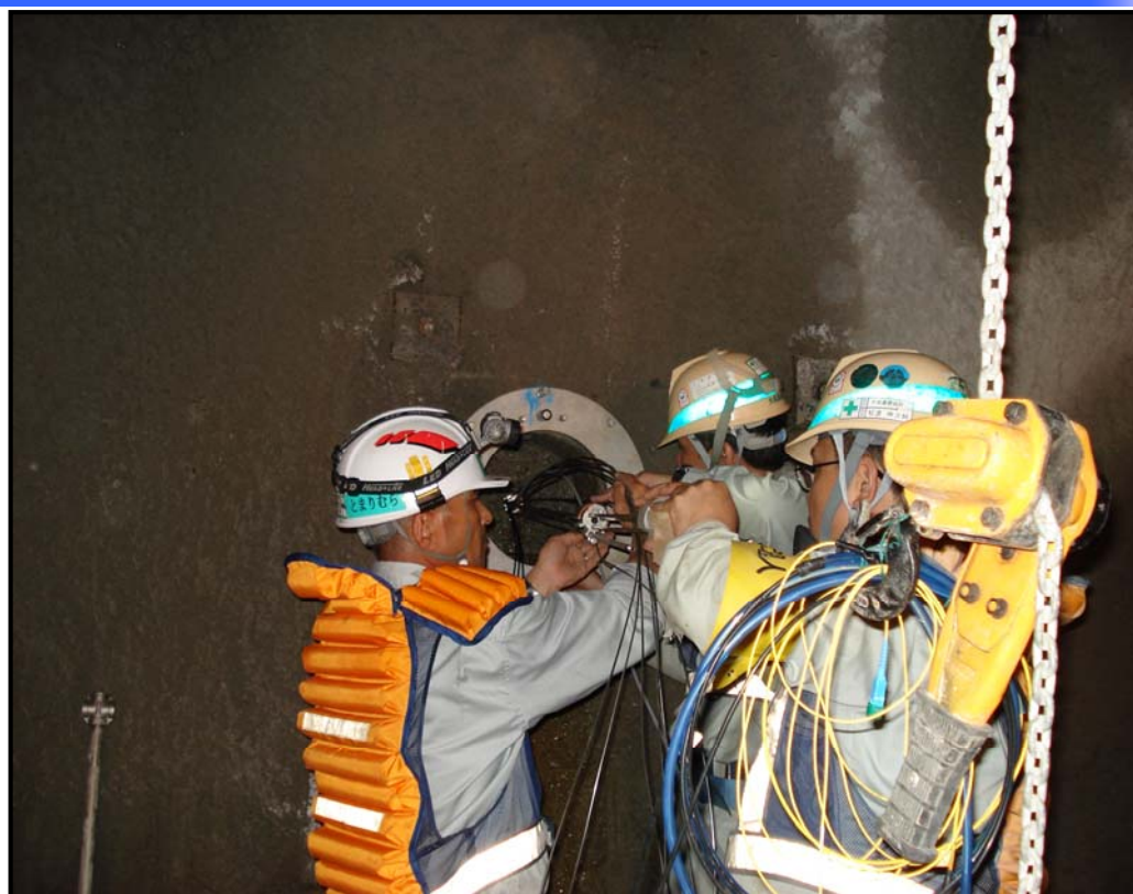
換気立坑：深度70m
