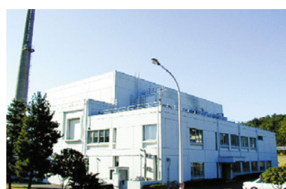
WASTEF建家外観
