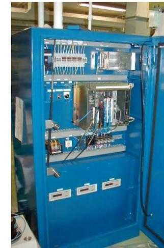
Sealed box including transformer of pressure to electric signal
