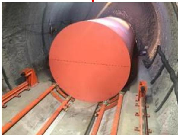
**PEM (Prefabricated Engineering barrier system Module)：**
