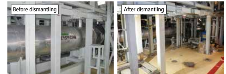
Heat exchanger of reactor core isolation cooling system for emergency
