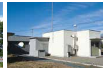
Takasaki monitoring station (measurement of particulates and noble gases)
