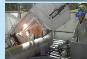
Dismantling of the control-rod drive mechanism casing
