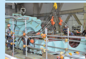
Current status of the dismantling of turbine generator
