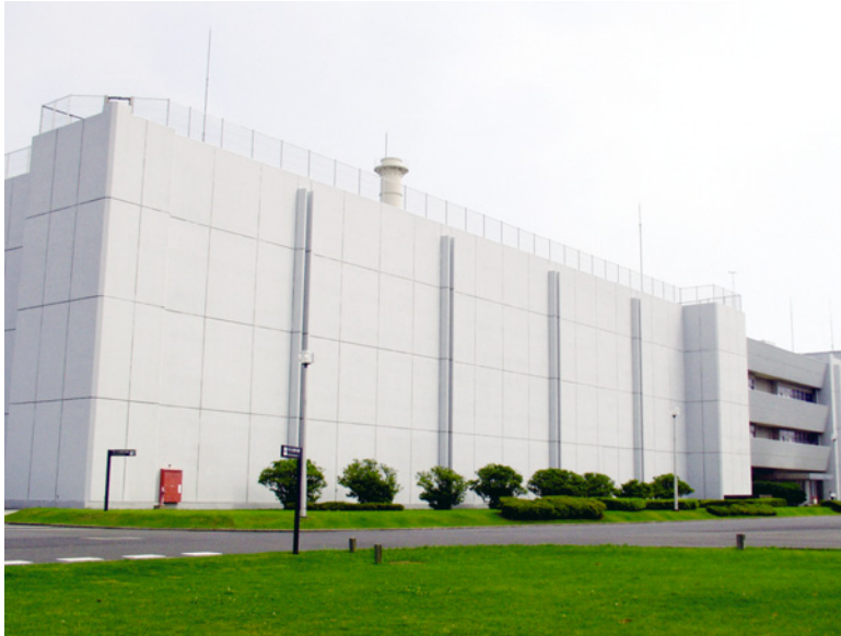
▲Overview of Plutonium Fuel Production Facility
