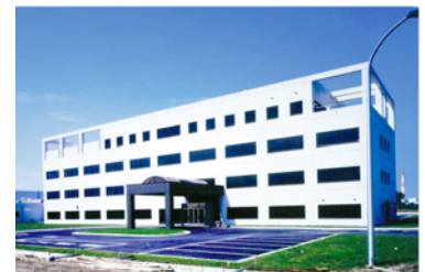
Completion of the Engineering scale Test and Research Facility
