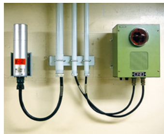
▲Area monitor (Monitoring of the working environment)
