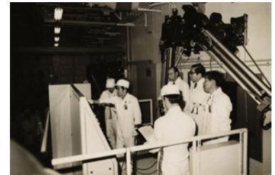
Start of test utilizing spent fuel at the Tokai Reprocessing Plant
