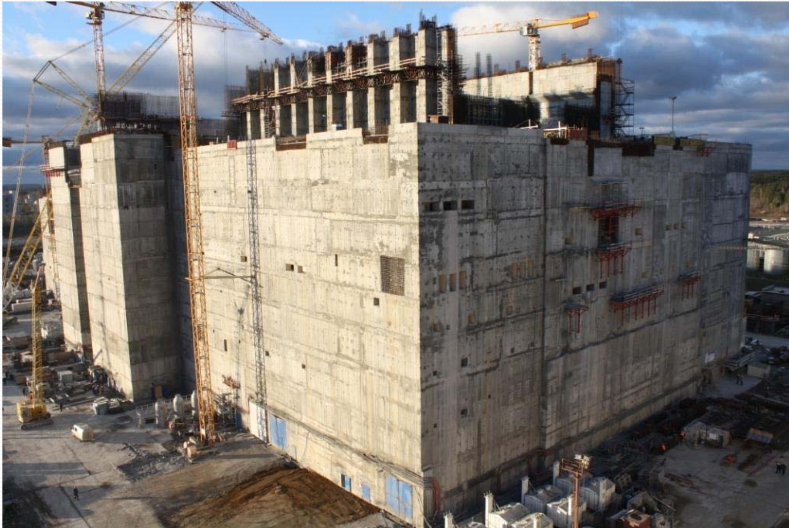
Bird's-eye view of the reactor compartment of the main building (30.10.2012)
