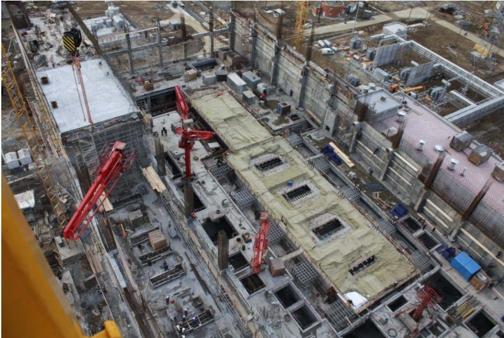
Bird's-eye view of the turbine hall. Concreting the turbogenerator basement (30.10.2012)
