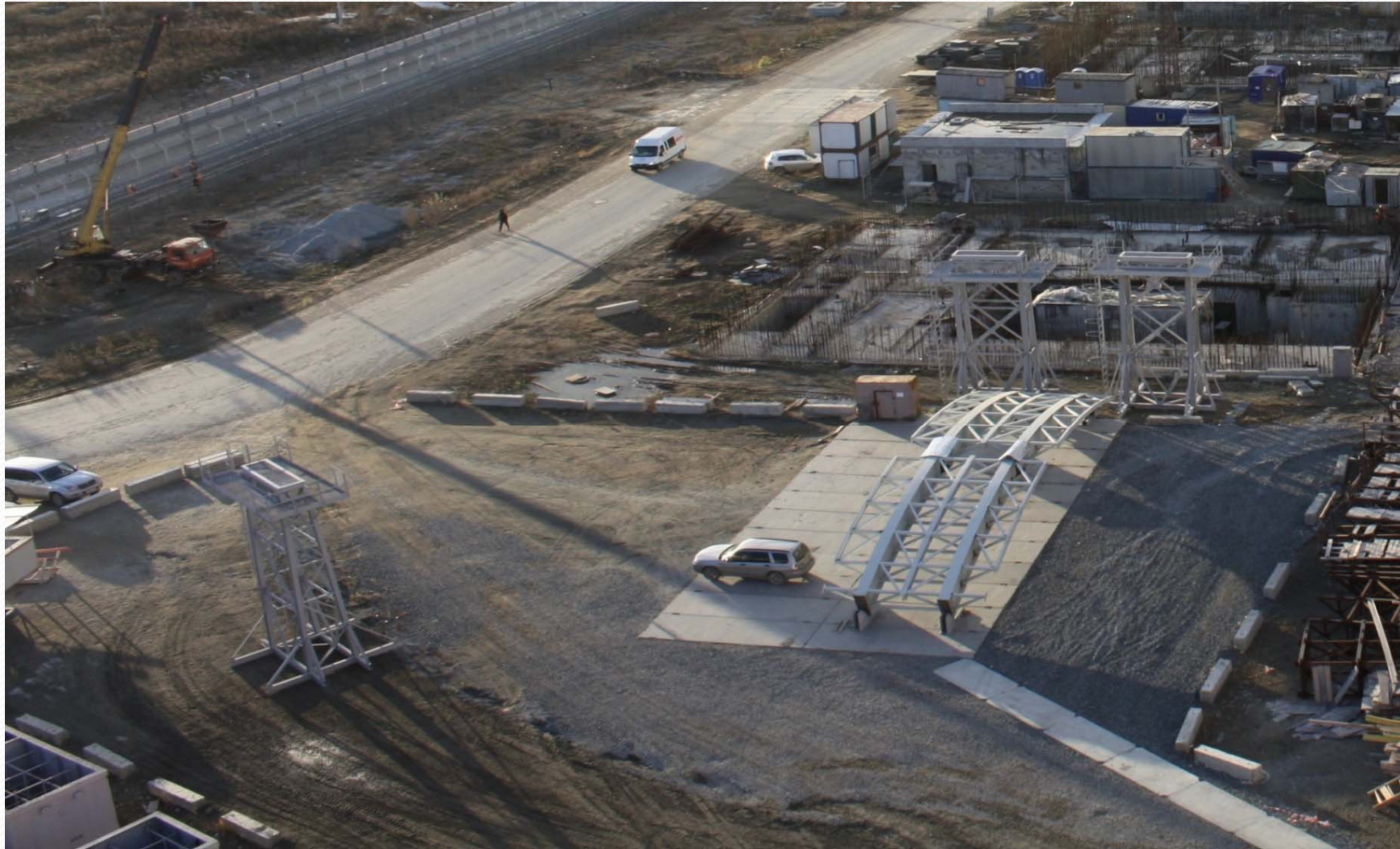
Bird's-eye view of the place for assembling metallic vault of the reactor compartment (30.10.2012)
