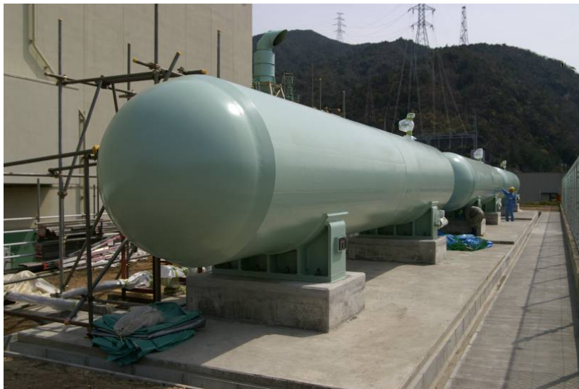
Installation of nitrogen tanks for Na fire extinguishing
