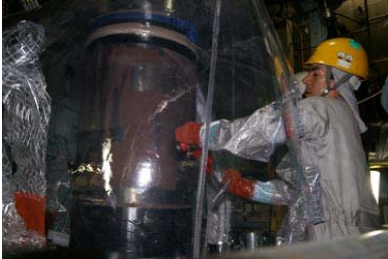
Replacement of temperature sensor
