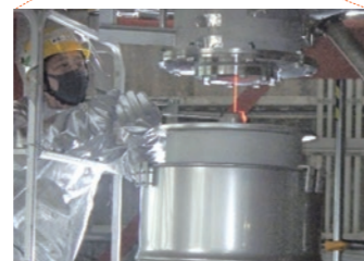
A bird's-eye view of the advanced melter (Upper) Glass pouring from drain nozzle in operation test (Lower)
