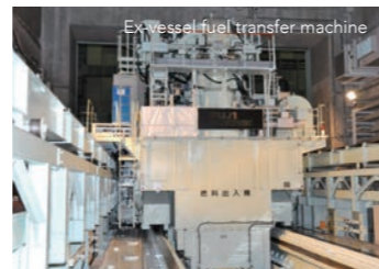
Fuel unloading operation at Monju
