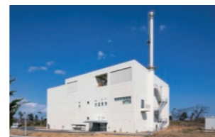
Oarai Waste Reduction Treatment Facility (OWTF)
