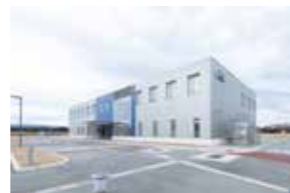
CLADS Main Building
