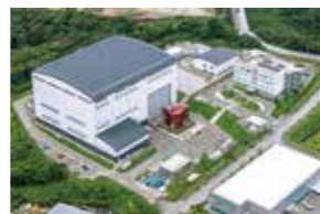
View of Research Management Building and Full-scale Mock-up Test Building
