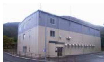
Sodium Engineering Research Facility (SERF)
