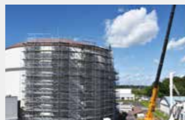
Seismic retrofitting work on JRR-3
