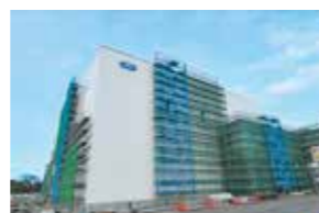
Construction status of Radioactive Material Analysis and Research Facility Laboratory-1
