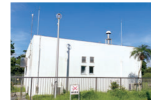
Okinawa monitoring station (measurement of particulates)
