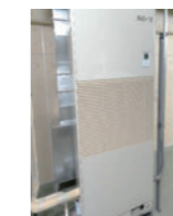
Efficiency improvement by renewing air-conditioning equipment
