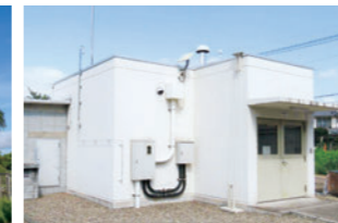
Takasaki monitoring station (measurement of particulates and noble gases)
