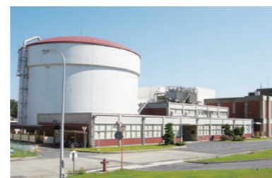
Research Reactor JRR-3
