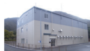
Sodium Engineering Research Facility (SERF)
