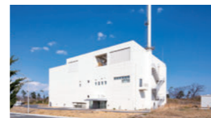
Oarai Waste Reduction Treatment Facility (OWTF)
