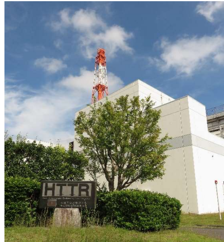
HTTR reactor building
