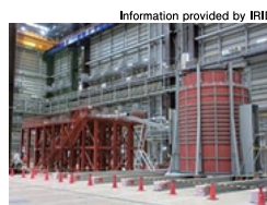
Full-scale mock-up testing facility for investigating the inside of PVC.
