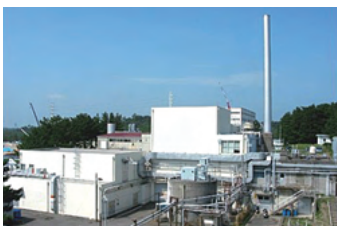
JRTF: JAERI Reprocessing Test Facility being decommissioned (Nuclear Science Research Institute: former JAERI)
