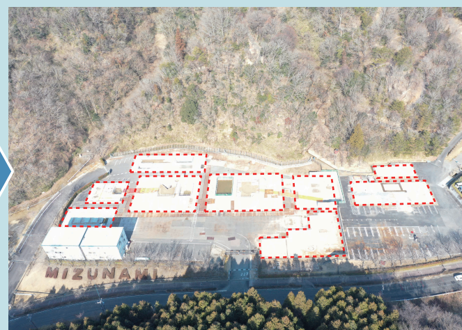
After demolition of the surface facilities (February, 2022)
