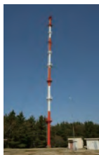
気象観測塔 Meteorological Observation Tower
