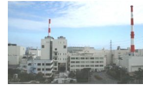
Tokai Reprocessing Plant
