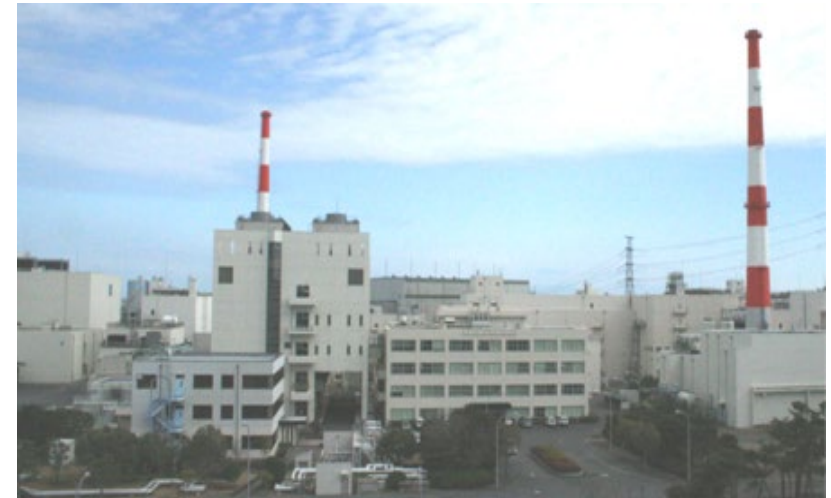
Tokai Reprocessing Plant
