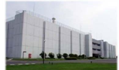
Plutonium Fuel Production Facility (PFPP, Pu-3)
