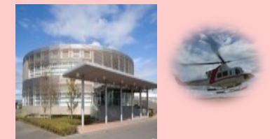
Nuclear Emergency Assistance & Training Center (NEAT)
