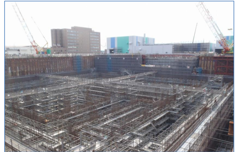
Progress of construction: 8.6% (September 2014)
